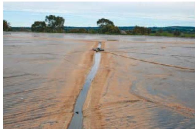
The sand weight that helps keeps the cover on the dam.
